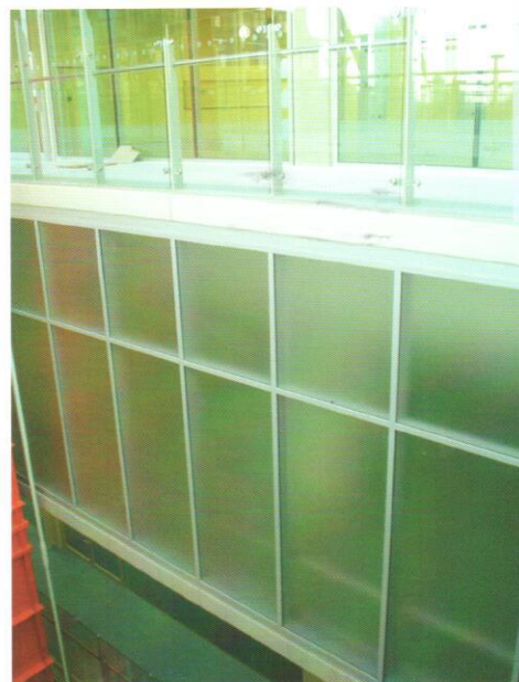
Evelina Children's Hospital, London: Sandblasted PYRAN® S offers privacy as well as reassuring safety.
